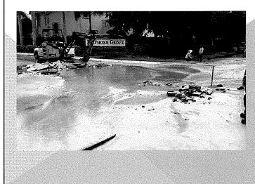
May 12, 2018, contractor for a wireless carrier installing fiber via directional bore struck a water main, which caused a flood and the road collapsed, creating a sink hole which blocked the entrance to a neighborhood in Cooper City. (Sun Sentinel picture)
