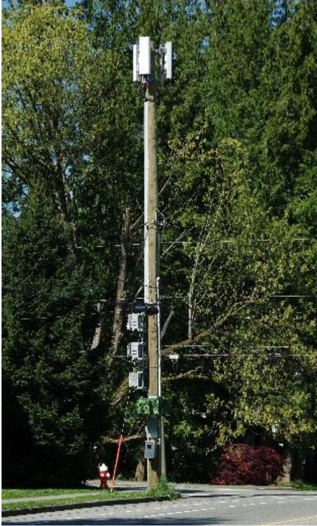
Exhibit 10. Wooden poles are prohibited. The City is transitioning away from wooden poles. In addition, the top-mounted antennas extend on arms away from the pole. This design is prohibited.
