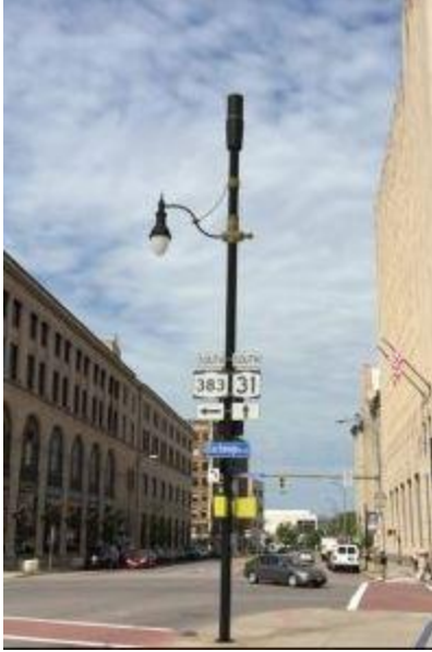
Exhibit 12. The pole lacks a base in scale to the volume of the antenna, which is larger than the diameter of the pole and does not appear to be an original part of the pole. This design would be prohibited.
