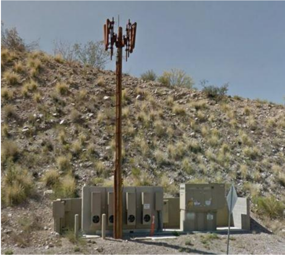
Exhibit 11. Antennas on arms are prohibited.
